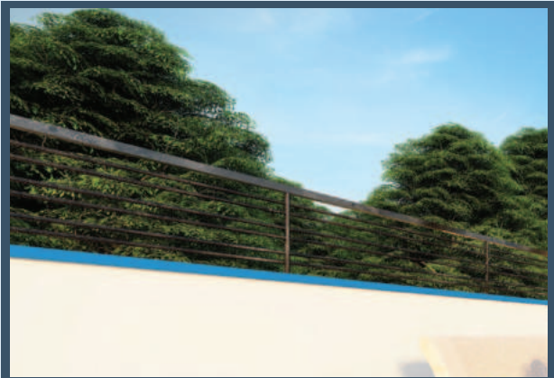
Outer Boundary Wall with Wire Fencing
